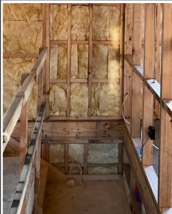
A midfloor 'ribbon' photographed half way up the stairs
