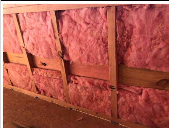
140mm blocking on edge to support flashing for the apron roofing – note that the remaining 45mm X 140 mm gap on the face remains uninsulated
