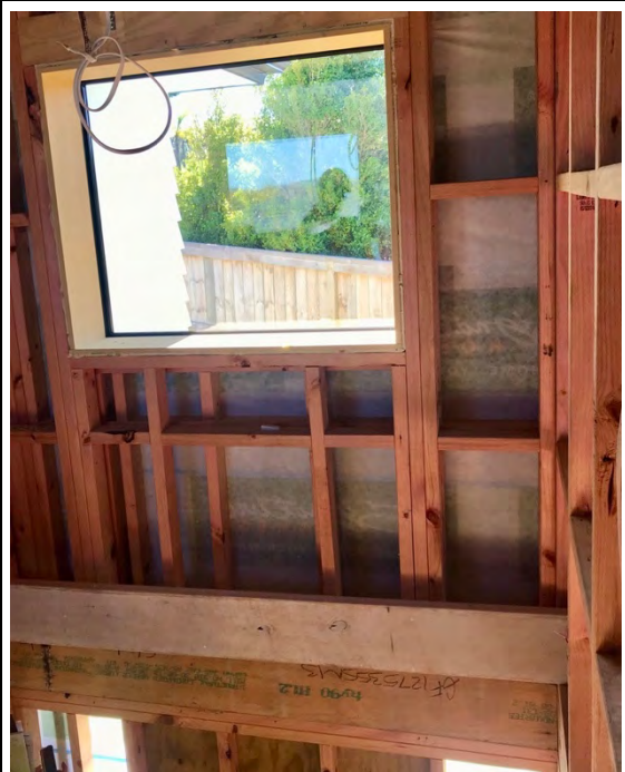
A midfloor junction in the open void of a large stairwell
