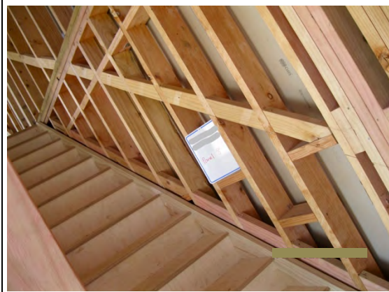
140mm blocking on edge to support flashing for the apron roofing – note that the remaining 45mm X 140 mm gap on the face remains uninsulated
