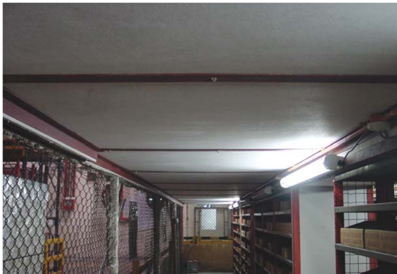
Above Installation of PROMATECT®-H suspended membrane ceiling at Chevron Phillips Cherrit International in Boon Lay, Singapore.
