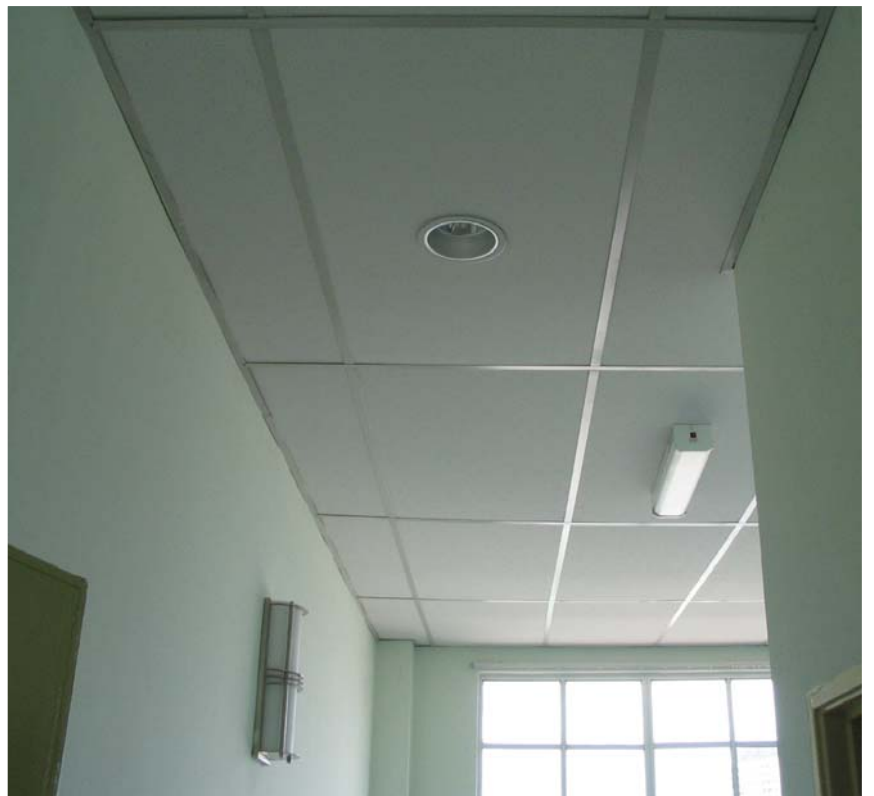
Opposite PROMATECT®-H integrity only suspended membrane ceiling at Hospital Pantai Ayer Keroh, Malacca, Malaysia.
