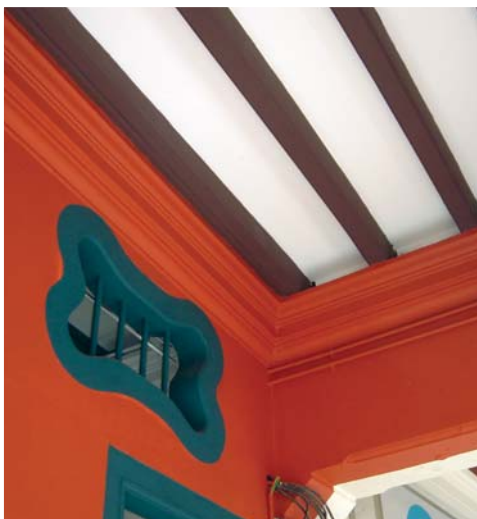
Below PROMATECT®-H 60 minute fire resistant timber floor protection for a heritage building in Beach Road, Singapore.
