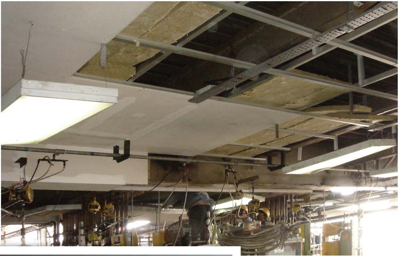
Above Installation of PROMATECT®-H suspended membrane ceiling at Chevron Phillips Cherrit International in Boon Lay, Singapore.
