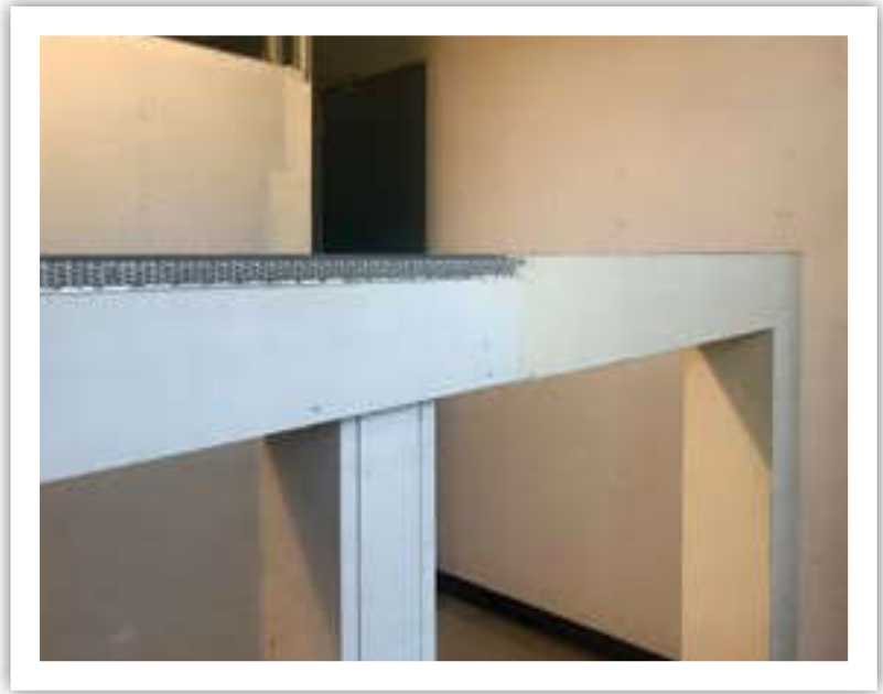
Plastering the board joints in structural steelwork and the partitions (on background of the picture).
