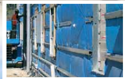
Heavy Gauge Top Hats Available in a range of sizes for fixing cladding to interior and exterior building structures.
