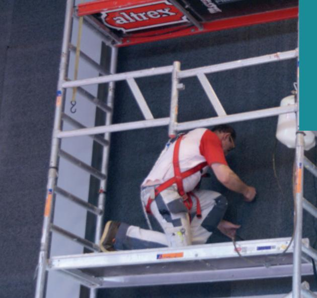
Arkema Cofix S is supplied in a canister of 25lt or about 20 kg. Apply Cofix S to both corresponding surfaces at a rate of 200 grams per square metre. Adhesive may be applied to surfaces with spray gun or brush. This is sufficient to cover 40-50 m2 of coverage by applying it on both bonding faces as a contact adhesive.
