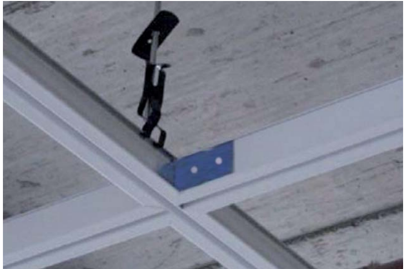
Clean mitred cross runner intersection.
