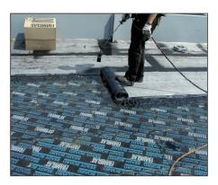
The upper surface of FOAMGLAS® Ready-Board is covered with a bitumen coating. A thin polypropylene film, which will burn off when a torch is applied. FOAMGLAS® insulation is ideal for roof over high moisture or high humidity - generating facilities.
