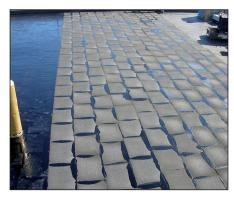
FOAMGLAS<sup>®</sup> is installed in hot bitumen on a continuous decking. The slabs are laid staggered with butted and bitumen filled joints. Quality of joint sealing easy to see. Install the roof membrane (BUR, Single-Ply or modified) in accordance with the membrane manufacturer's recommendations.
