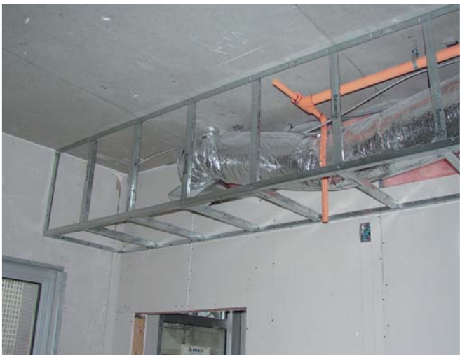
Right: QuikStix Bulkhead Installation in progress
