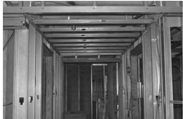
Corridor framing using traditional steel studs
