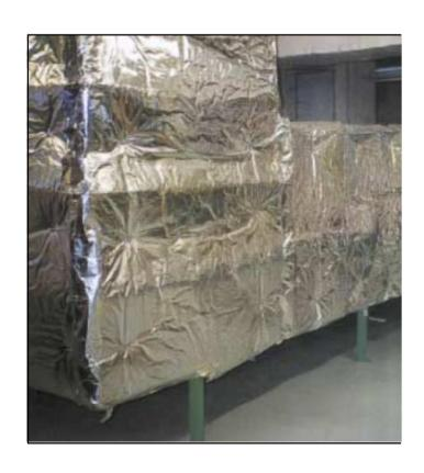
Ducts of larger dimensions should have Ductwrap applied with a minimum of 50% coverage of fire rated contact bond adhesive to all sides of the duct. Impale Ductwrap over mechanical fasteners (spot welded or adhered pins) at a maximum of 450mm centres.
