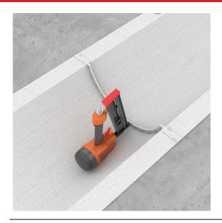
Fold the 50mm lap in half then staple together with another row of staples at 50mm centers using a pneumatic staple gun and 12mm FIREFLY stainless steel staples.
