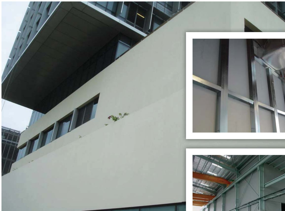
Clockwise from above: PROMINA®-HD external wall claddings at Khoo Teck Puat Hospital in Yishun, PROMATECT®-H steel stud partition at New Tech Park and PROMINA® 60 external wall claddings at a warehouse in Gul Road. All projects in Singapore.
