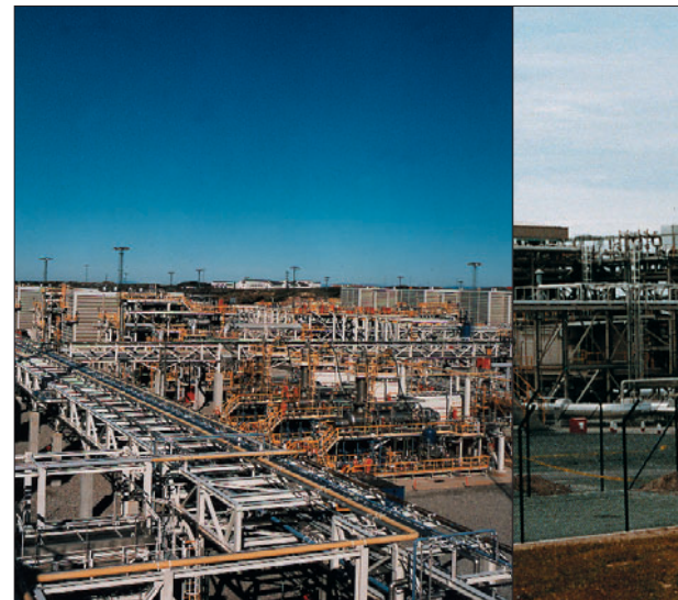
Troll Gas treatment plant at Kollsnes.
