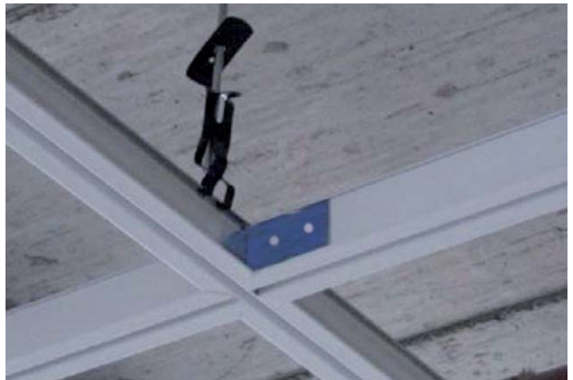
Clean mitred cross runner intersection.
