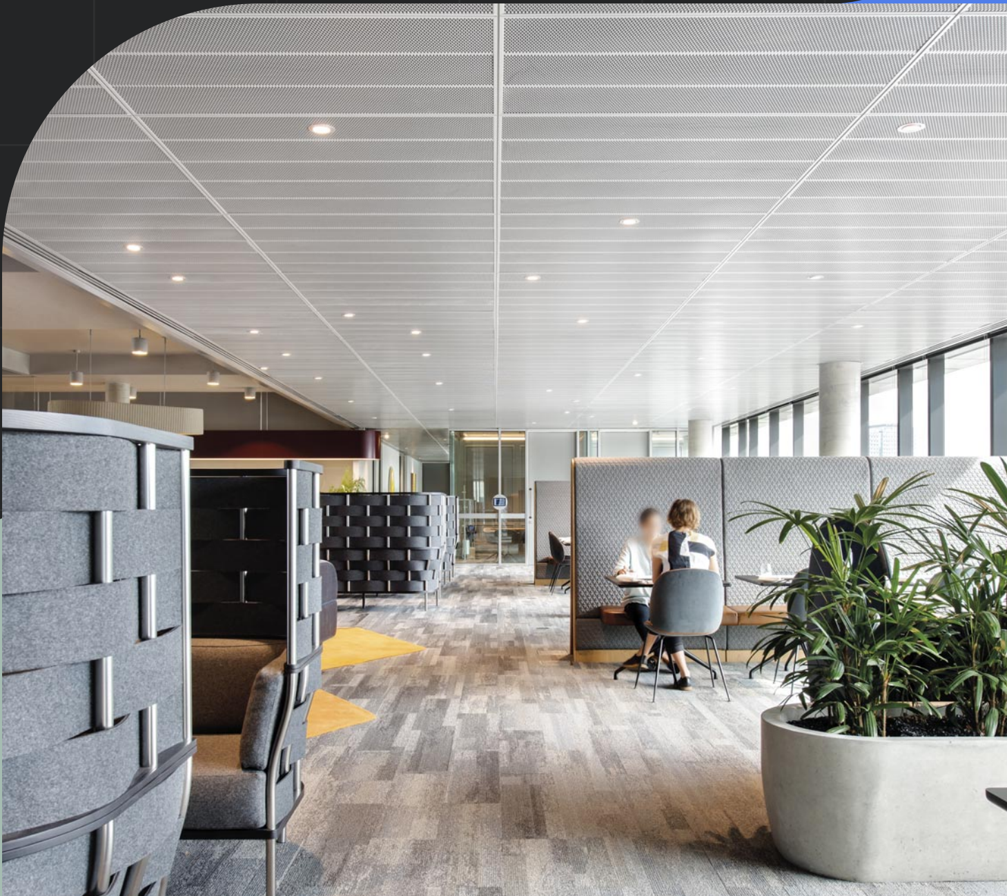
Image: METALWORKS One Way Hook On Ceiling installed at PWC offices in Melbourne, VIC
