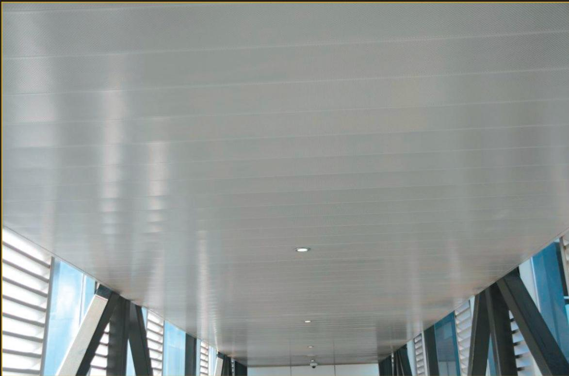
HARMONI 180 is an elegant ceiling system that can be used in a broad range of applications. The 180mm wide monolithic panel provides a wider concealed fix system that gives greater focus to the ceiling plane whilst retaining plenum access. HARMONI 180 is equally effective in small and large spaces and has a non-woven bonded acoustic backing which delivers premium acoustic performance.
